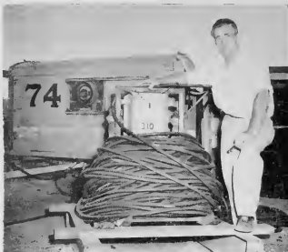
R. MacMillan won Fls. 150 for his idea of mounting Portable welding stands on pallets. MacMillan is shown above standing beside a palletized stand which
